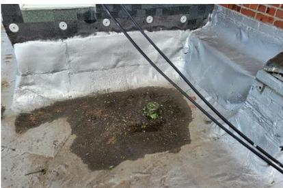
*The storm ripped up the flashing on the roof*
